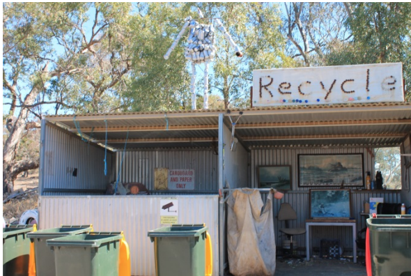
Recycling centre, Coolah
